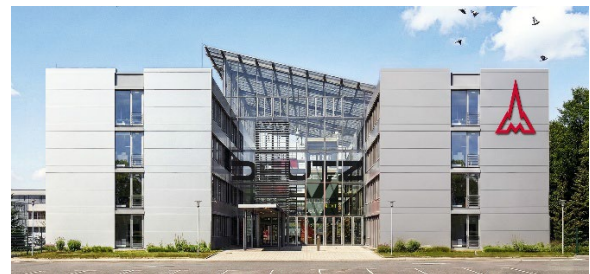
Caption: The new word and figurative mark at the headquarters in Cologne-Porz.
